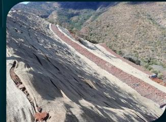
**Top:** Erection of a gabion toe line during the construction phase **Bottom:** The finished product showing erosion control channels and blankets in Dublin Asbestos Mine in Mafefe Village, Limpopo Province.
