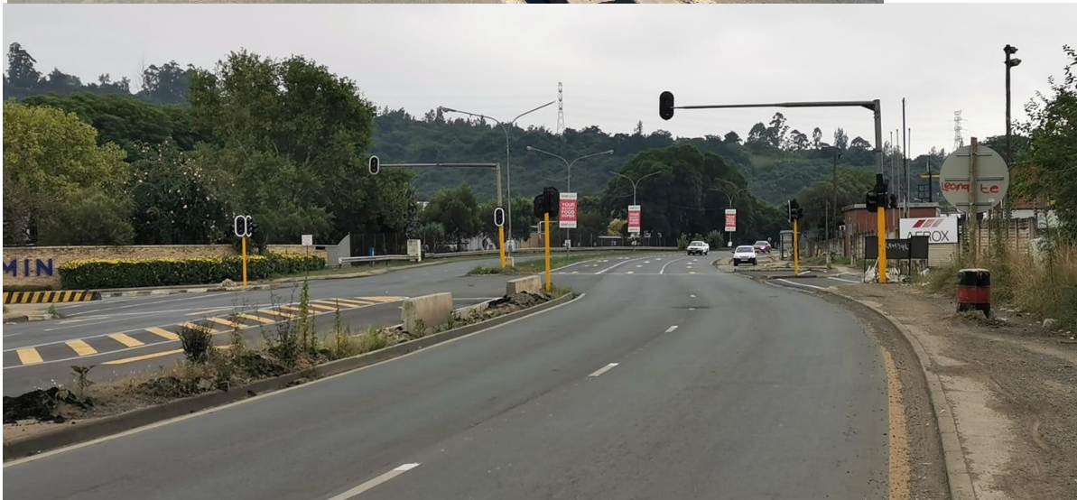
Lanes for resurfacing along Hulamin
