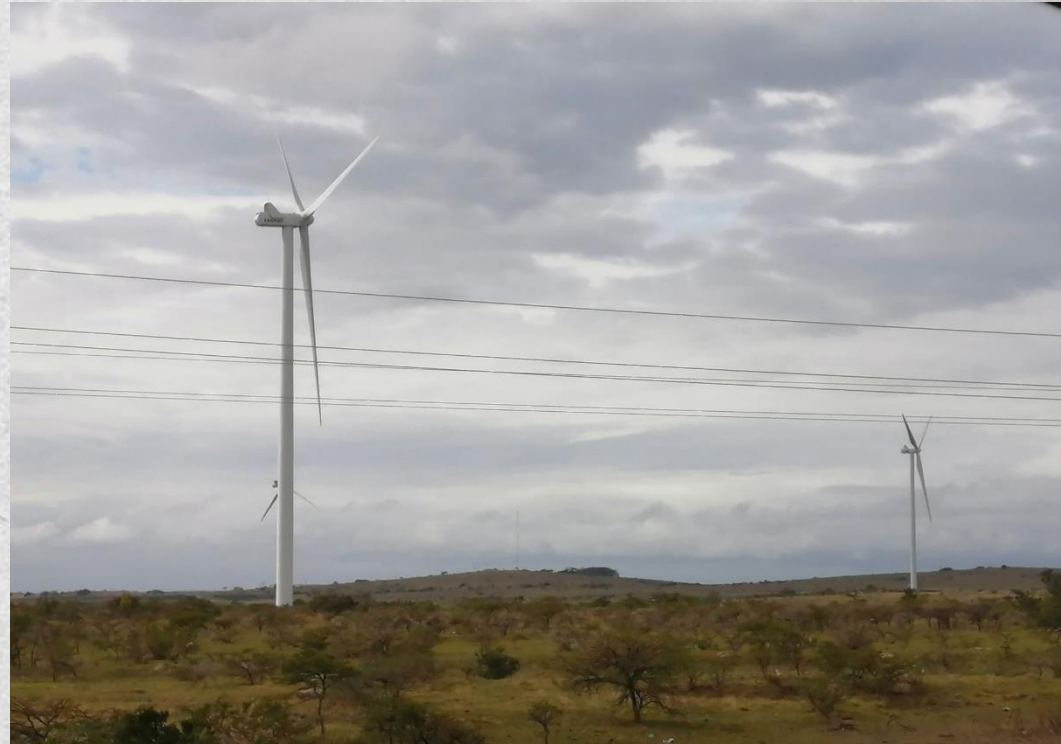
Latest wind farm commissioned in the Eastern Cape - Wesley
