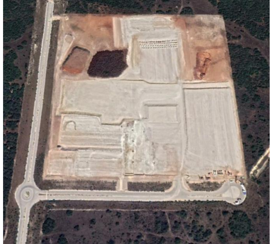
Tank Farm site - Bulk Earthworks
