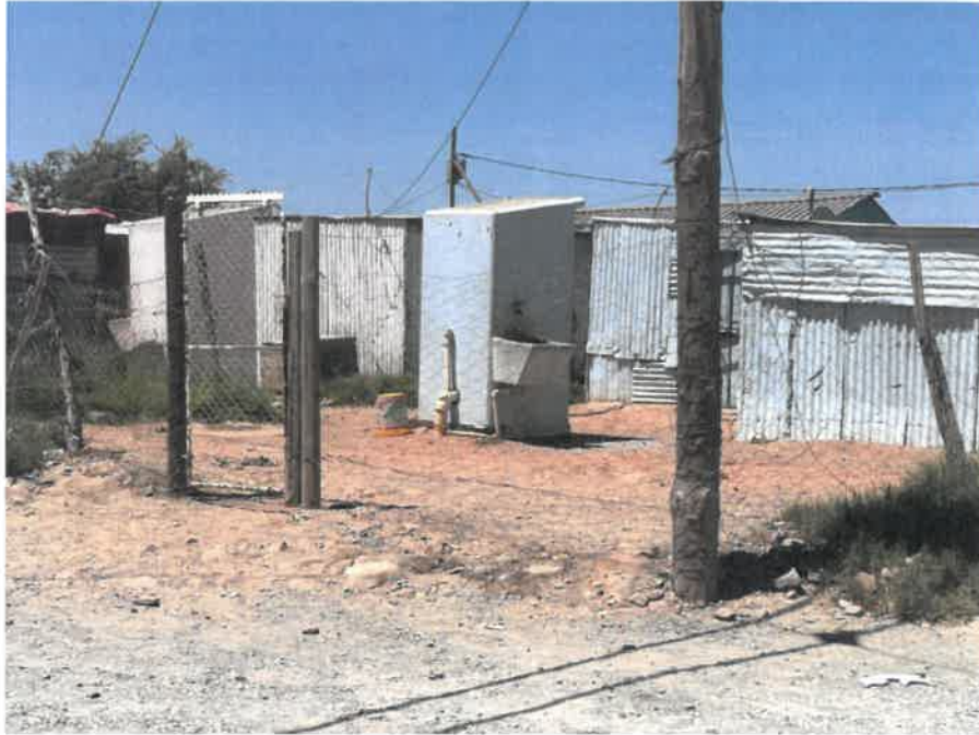
Picture 2: Enhanced Service site wet core structure.
