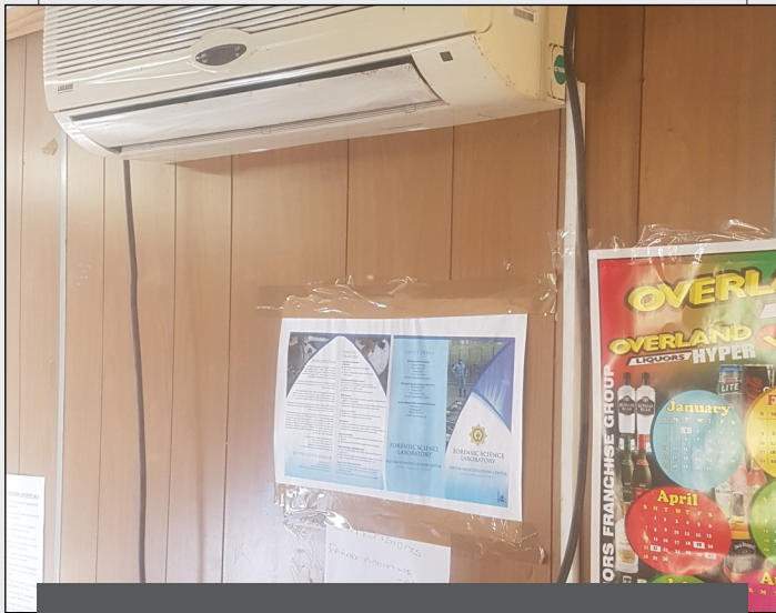
Boitekong satellite police station was found to be of poor quality
