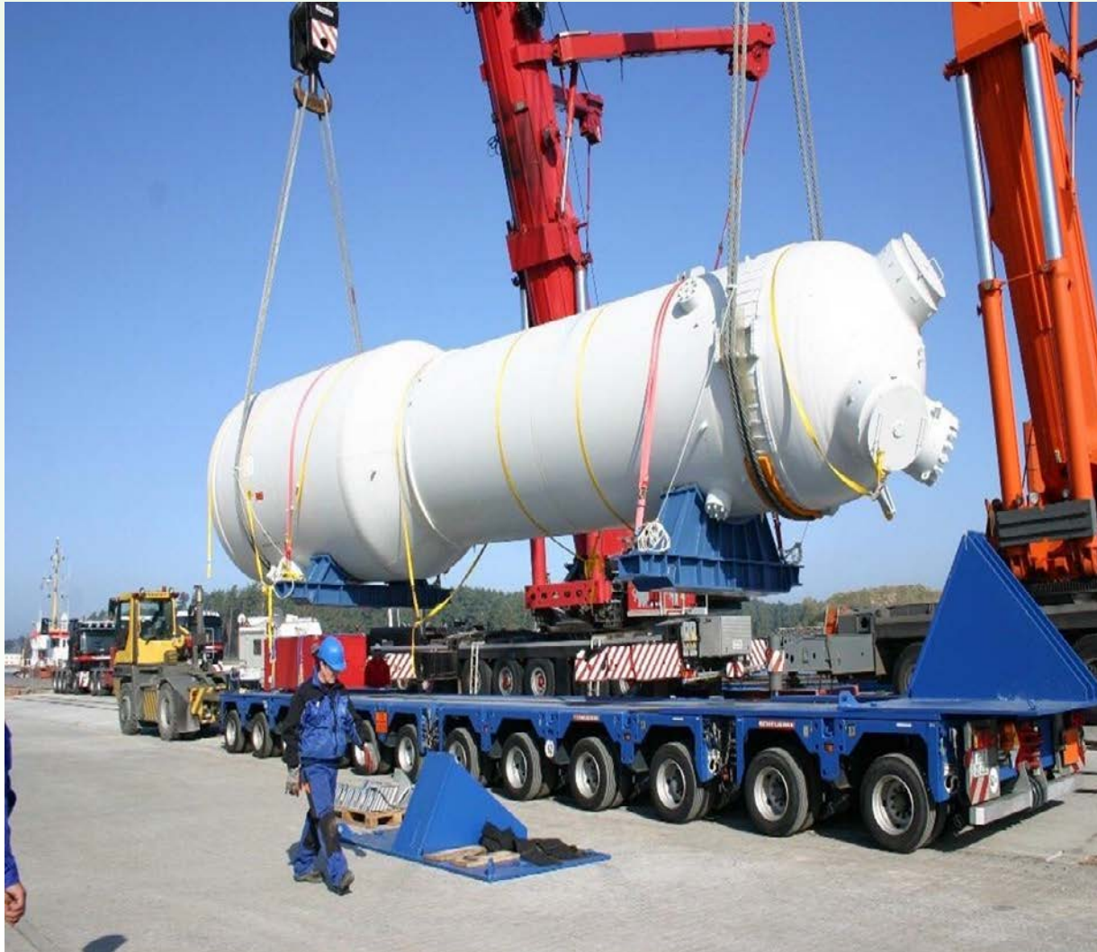
ORIGINAL STEAM GENERATOR
