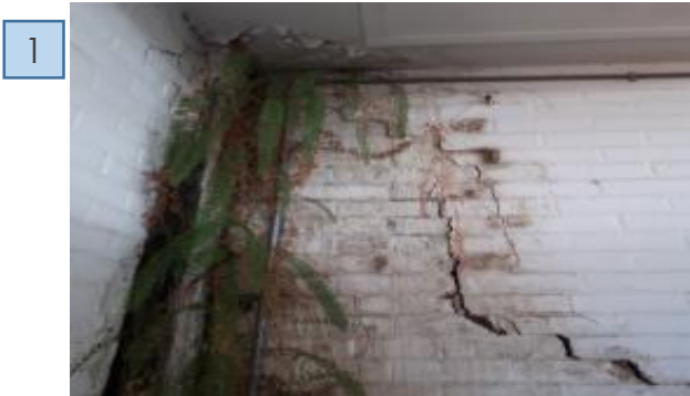
Picture 1: Structural crack and plant encroachment (GP) at Chris Hani Hospital
