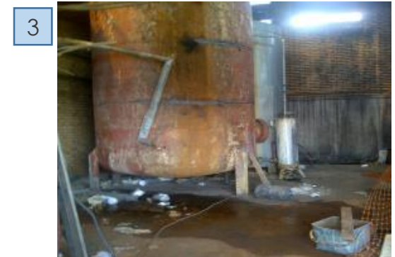
Picture 3: Leaking boiler (GP) at ODI Hospital
