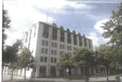
Police Station Munich-Schwabing
