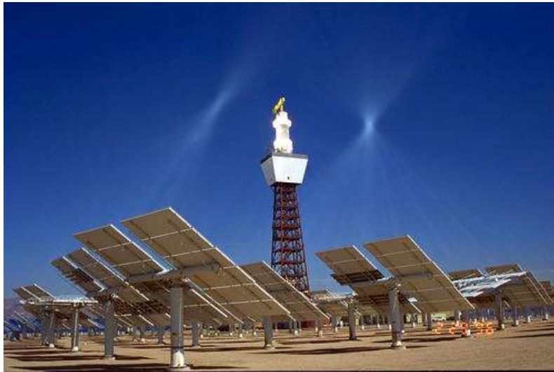
Figure 6-24 Picture of Central Receiver Plant
