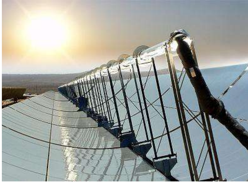
Figure 6-22 Parabolic Trough North-South Axis View
