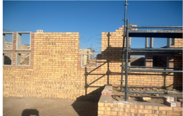
Ground floor wall plates with window frames
