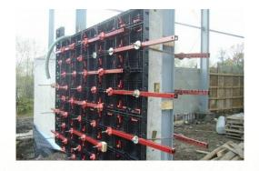
GeoPanel Formwork System is a temporary shuttering system for the construction of concrete walls, columns and beams. It consists of a series of various sized panels joined together by the Geoplast fastlock nylon handle. The formwork system is made of acrylonitrile-butadiene-styrene (ABS) polymer and other additives (pigments, polymer additives, antioxidants, and colourants).
