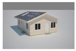
**Besta Board Building** System is a singlestorey structure that utilizes factory produced Fibrous Magnesium Oxide (MgO) boards and a light-weight steel superstructure that is sub-supported with a hot-dipped galvanised light-gauge steel frame.
