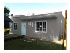
Polyform Building System consists of expanded polystyrene (EPS) modules with a density of 12 kg/m3, forming a central core of which is filled with (reinforced) concrete of 25 Mpa. The modules are finished with 15 mm thick plaster both sides.
