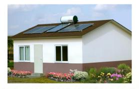
**Boen Eco Solutions Building System** is constructed with prefabricated components that are assembled on site. It utilizes conventional concrete foundations and a 100 mm thick surface bed which are always the responsibility of a registered competent engineer.
