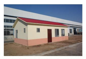
Shouguang Prefabricated Building System. The steel frames are manufactured from 78 mm x 1.2 mm thick hot-dip galvanised steel. The external and internal wall panels are tongue and groove steel edges consisting of 6 mm fibre cement boards on both sides encapsulating foam cement with a density of 517 kg/m3.
