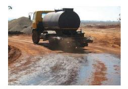
Ecobond, a non-traditional soil stabilizer, is a modified bitumen emulsion polymer. It is used for stabilizing road base construction materials for both paved and non-paved gravel roads as well as in wearing course for gravel roads.
