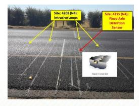
Mikros Dual Stick-on Loop Traffic Monitoring System consist of a dual stick on loop, RAKTEL X010/20, MICROSAC Card, RAKMAN Power Manager Card, TELOOP8-100 Loop Card, Battery, Bituthene 5000 or similar tape and GPRS modem to download data (optional). Permanent Dual Traffic
