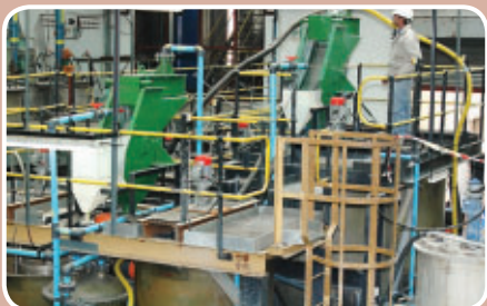
Uranium Pilot Plant at Mintek.
