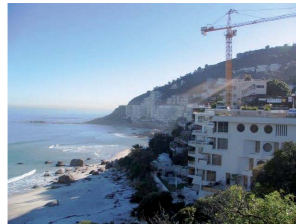
Construction site on prime land, Cape Town. Photo DAG
