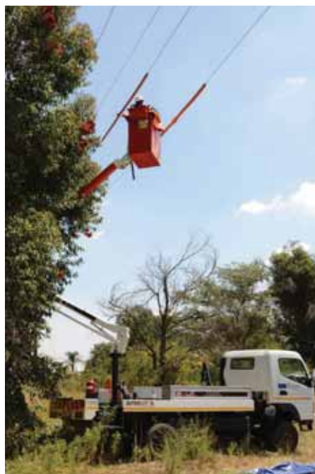
The Cullinan technical services team fixes a distribution line
