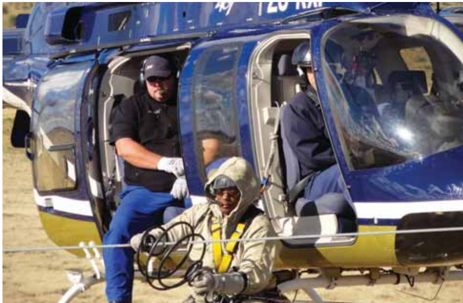
Bird diverters are strung on high-voltage power lines by helicopter
