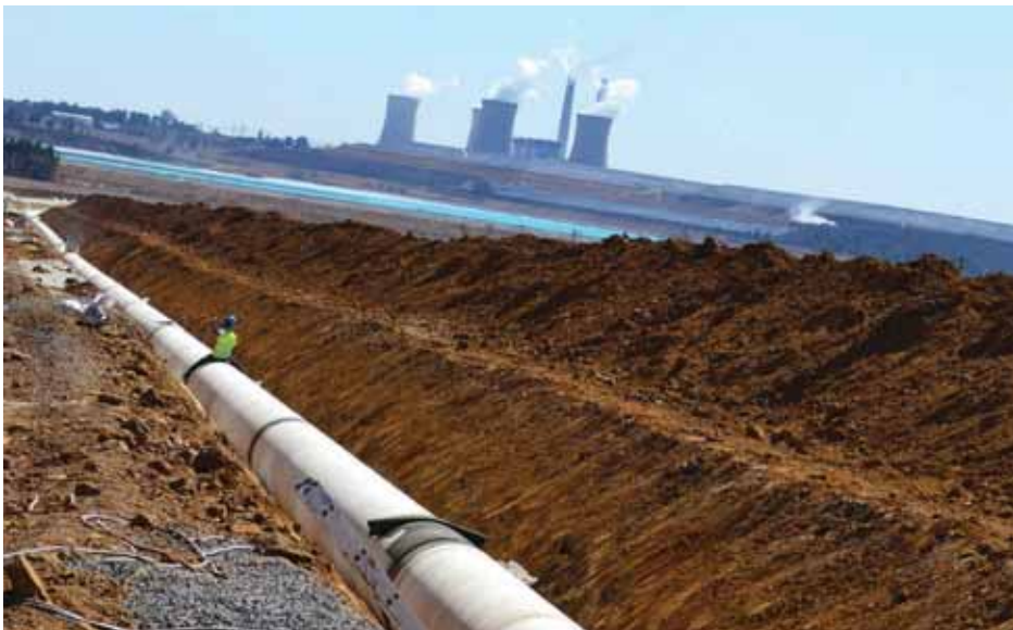
Construction of the new Komati water scheme
