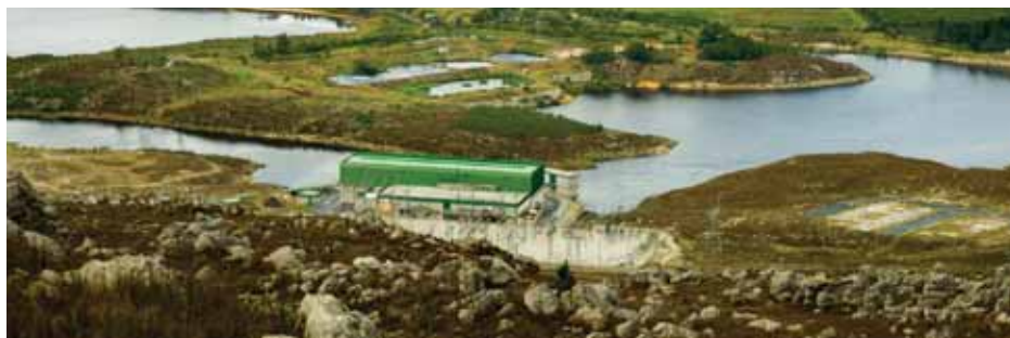
Palmiet pumped-storage scheme in the Western Cape is a joint venture between the Department of Water Affairs and Eskom, transferring water between the Palmiet and Steenbras Rivers for delivery to Cape Town
