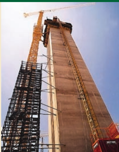
Medupi power station under construction
