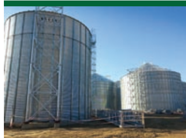
A STATE-OF-THE-ART SOYA BEANS CRUSHING PLANT IN MPUMALANGA
