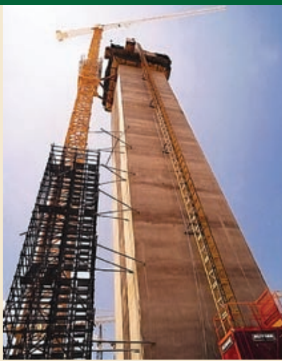
Medupi power station under construction
