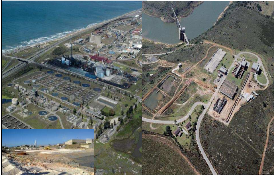
Water Treatment Works: Elandsjagt
