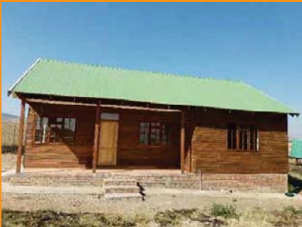
Vriesland Primary School Kitchen
